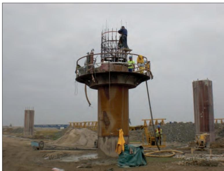
*Installation of O-cell test pile*
